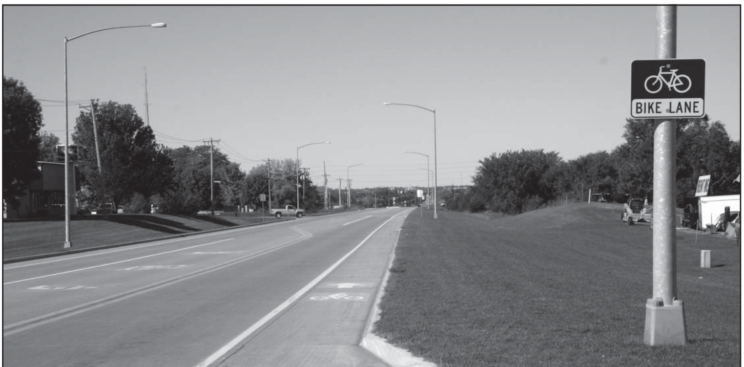
Well-marked bicycle lanes improve travel safety for bicyclists on this high-speed arterial roadway in Ames (photo courtesy of Bradley Grefe, CTRE at ISU).
