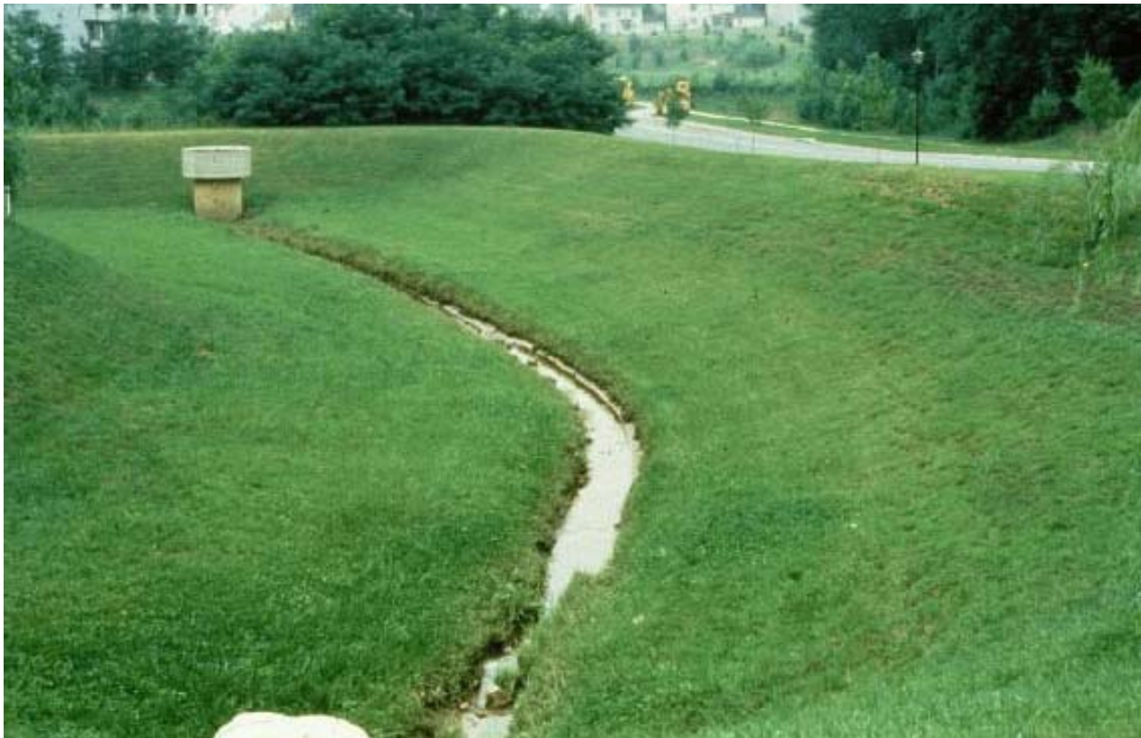
Figure 1: Dry detention basin
