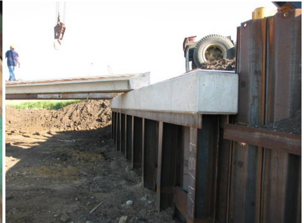
(b) Abutment cap on abutment piles
