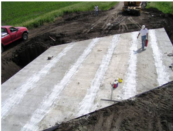
(e) Completed bridge without guardrails
