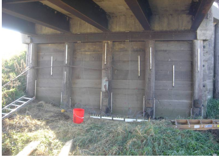
Figure 2. Timber substructure instrumented with strain gauges (south abutment, Bridge No. 237350, Mahaska County)
