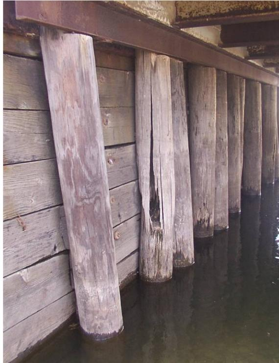
**Figure 1. Timber pile deterioration**
