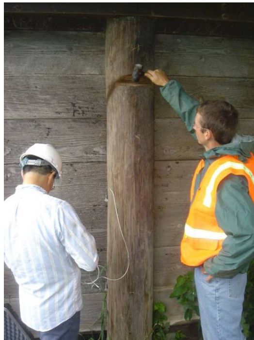
Figure 3. Pile integrity testing (Bridge No. 237350, Mahaska County)
