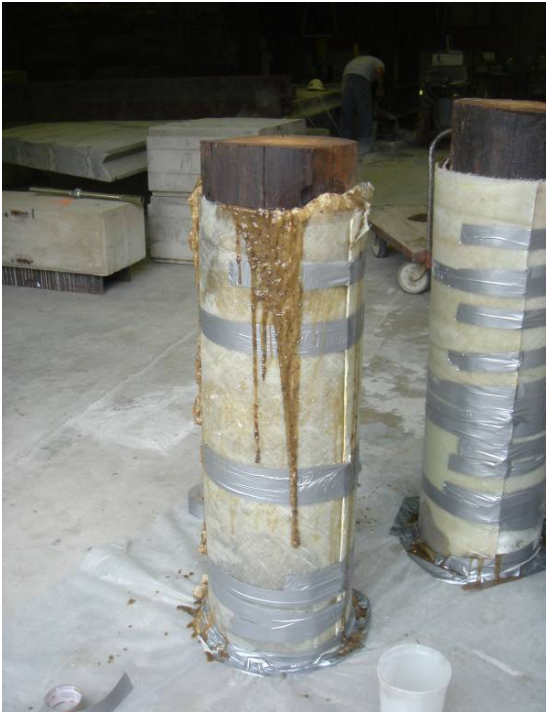
Figure 5. Timber pile repaired using filler epoxy and fiber-reinforced polymer
