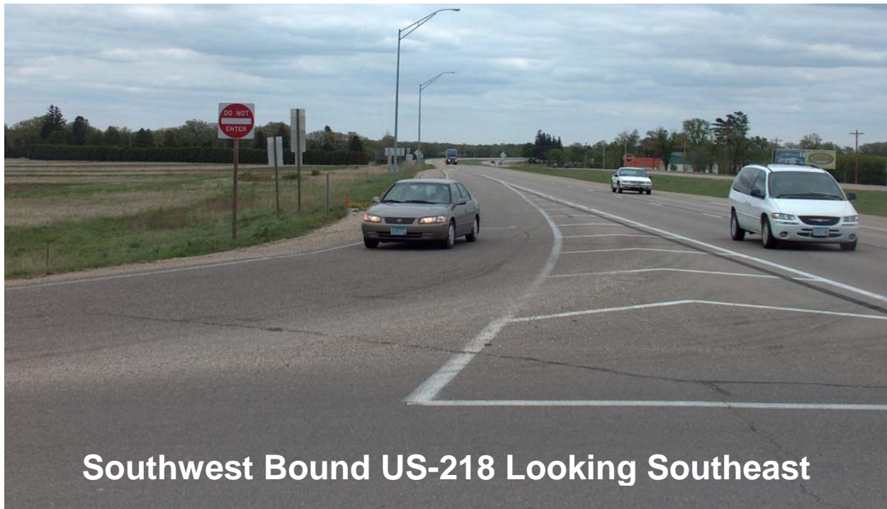
Figure 7. Offset right-turn lane at west junction of US-18 and US-218, Floyd, IA
