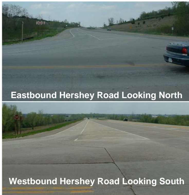
Figure 5. Offset right-turn lanes installed at US-61 and Hershey Road, Muscatine, IA
