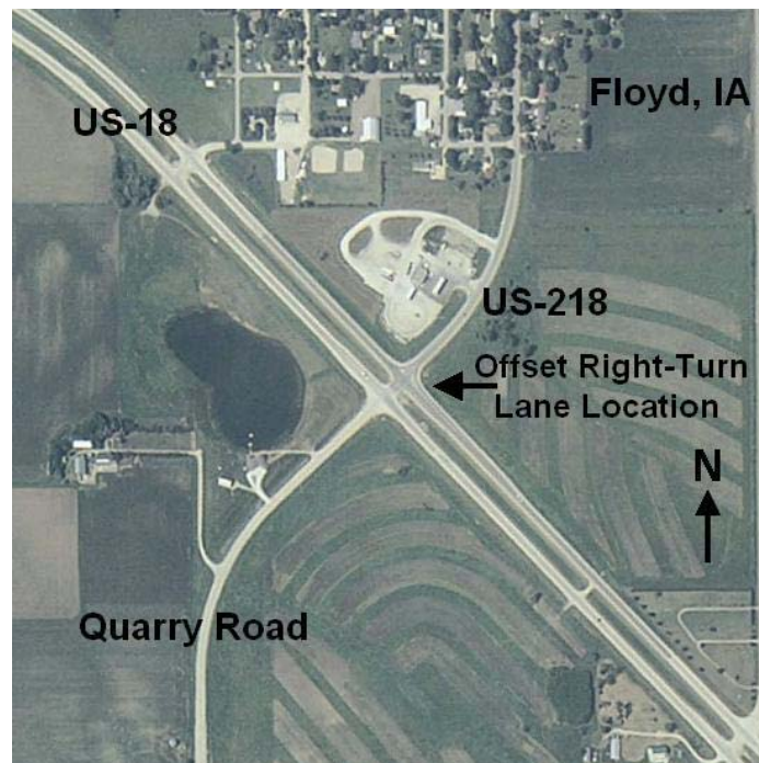
Figure 6. West junction of US-18 and US-218, Floyd, IA
