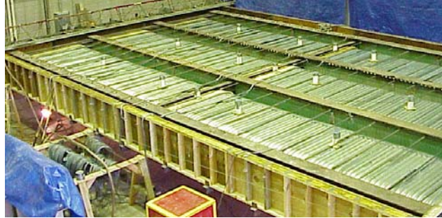
Figure 5. Installed modifications prior to the deck placement
