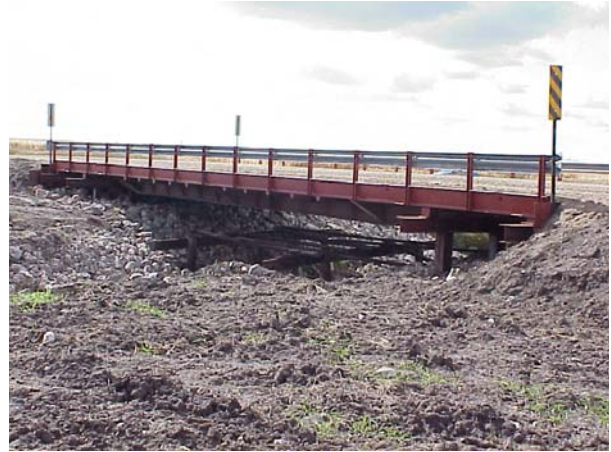
(b) Winnebago County Bridge
