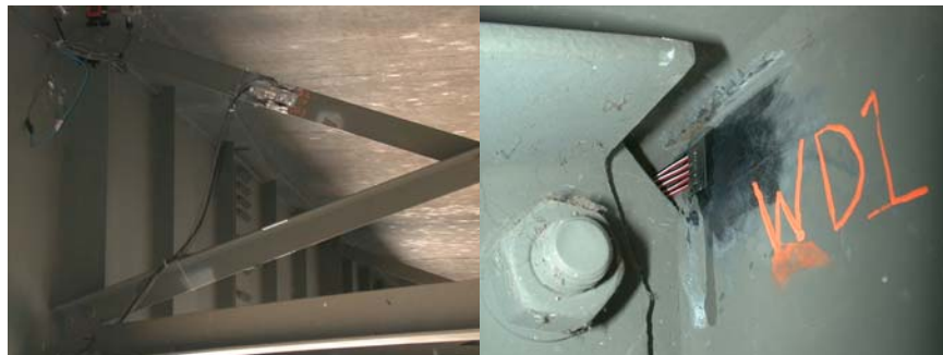
FIGURE 7. Photographs of Diaphragm and Web Gap Strain Gages
