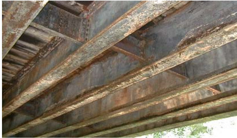
FIGURE 2. Photograph of Bridge Superstructure
