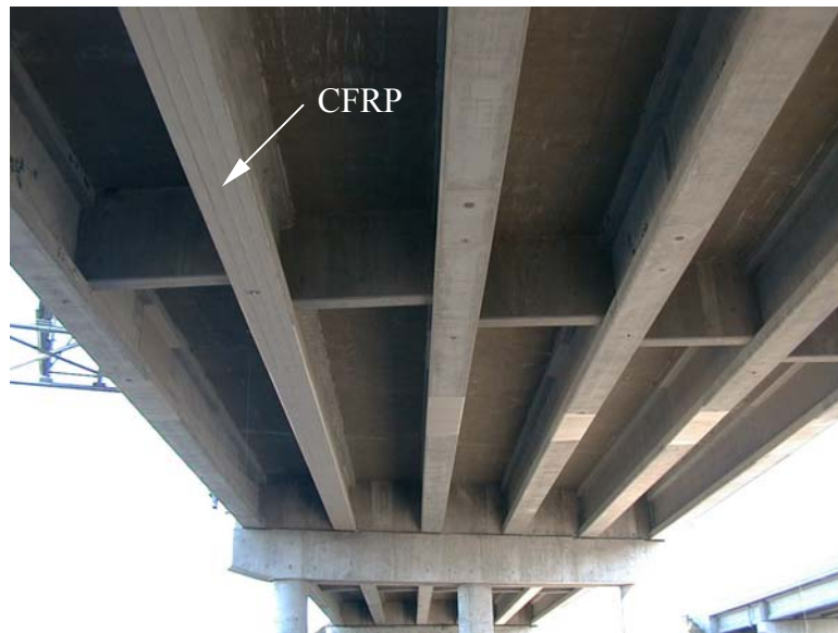
FIGURE 4. Photograph of CFRP on Beam 2 of Altoona Bridge
