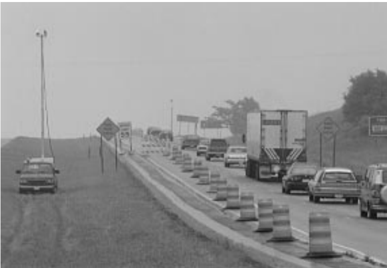
CTRE is collecting data on traffic/driver behavior in existing work zones. These data provide the basis for an Arena-based work zone simulation model.
