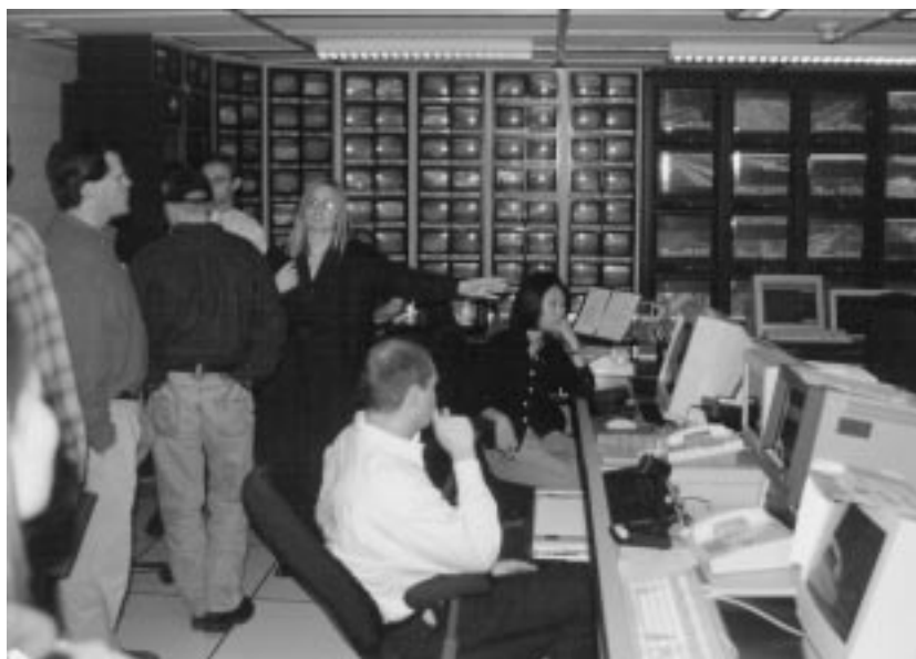
TSA members saw how MnDOT's Traffic Management Center monitors traffic flows at different locations in the Minneapolis/St. Paul freeway system.
