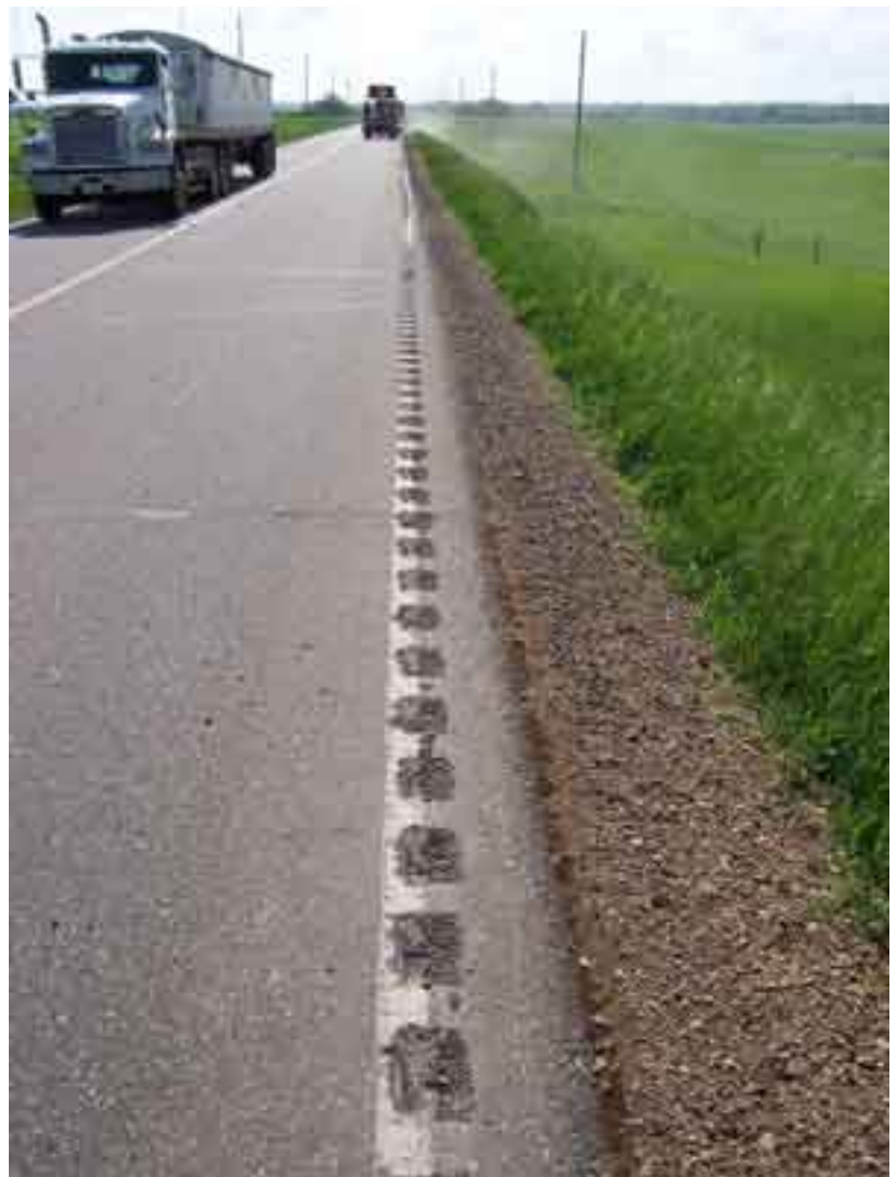
Milled-in rumble stripes soon be painted over with edge line
