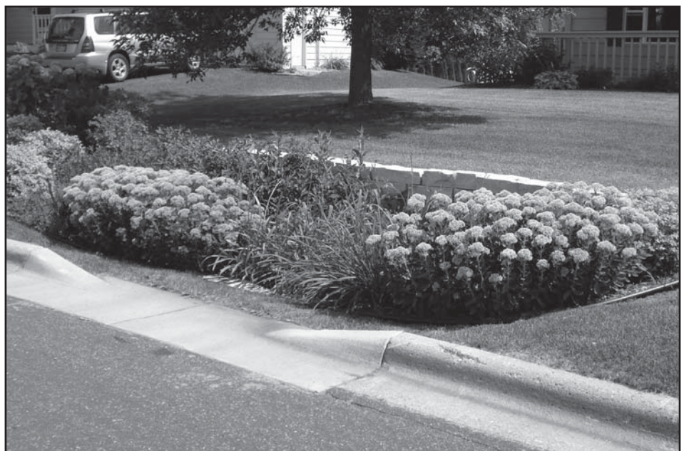
A rain garden is a flexible and aesthetic solution where a landscaped area collects surface runoff and then filters it through a variety of plants and a specially engineered soil mixture (photo courtesy of NRCS).
