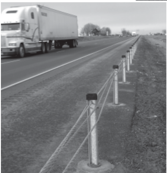
Four cables absorb energy from an impact. Photos courtesy of the Iowa DOT.
