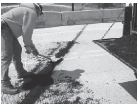
Rubber particles are spread and then sealed into the expansion joint. Photo courtesy of the Iowa DOT.
