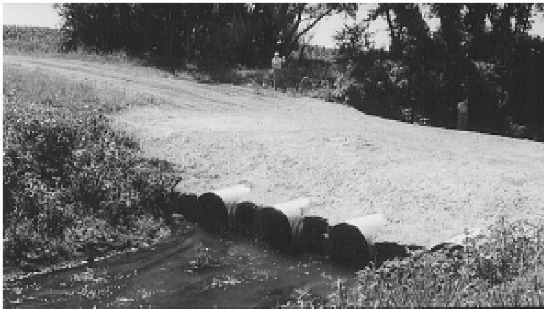
Vented ford with pipes (Tama County, Iowa)
