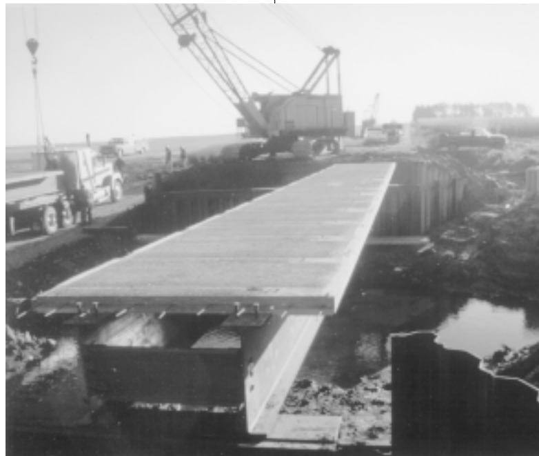
The precast units were set in place quickly.
