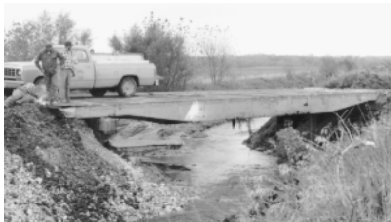
Construction of the Tama County RRFC bridge. Photo courtesy of the Tama County engineer's office.
