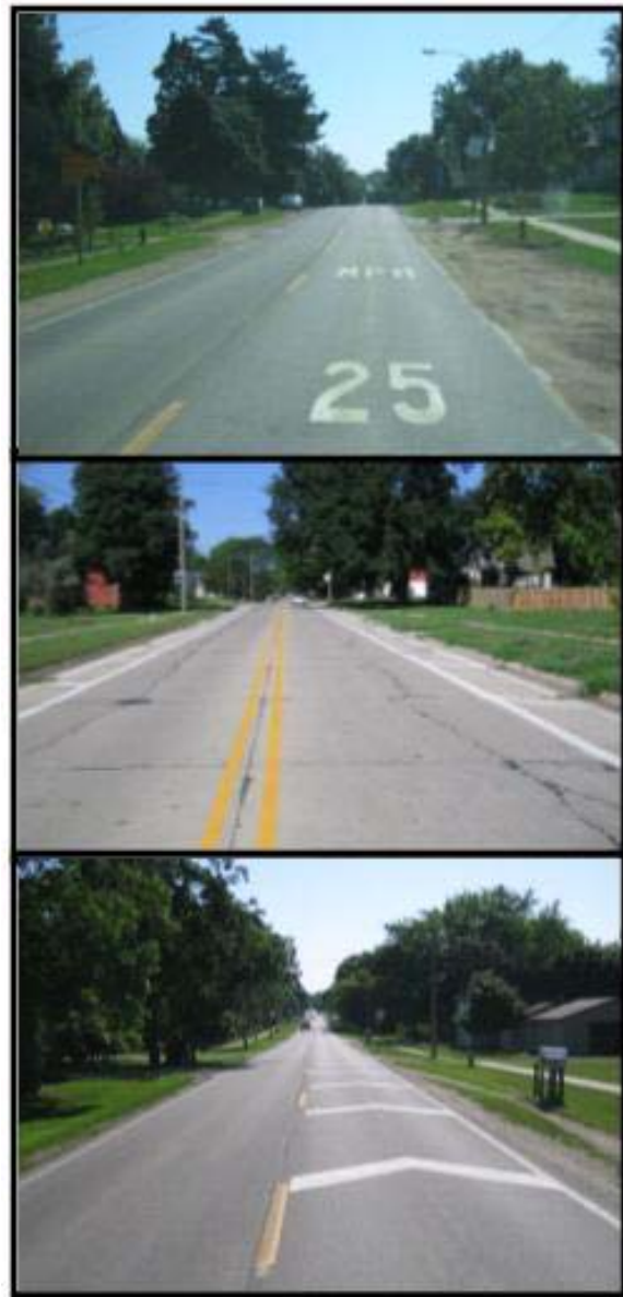
Figure 4: Roland, IA, after traffic calming (pavement speed signing, lane narrowing, converging chevrons)
