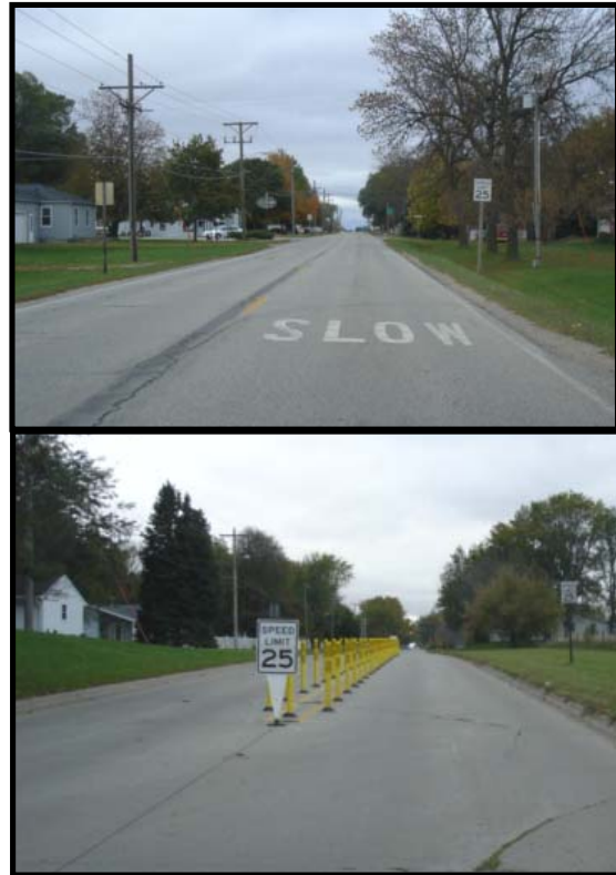
Figure 6: Slater, IA, after traffic calming (surface treatment, longitudinal channelizers)
