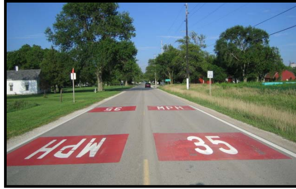
Figure 2: Dexter, IA, after traffic calming (surface treatment)
