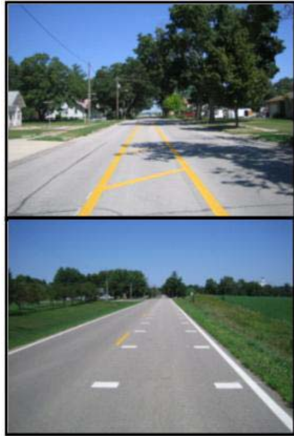
Figure 8: Union, IA, after traffic calming (lane narrowing, transverse bars)
