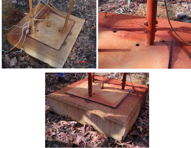
Figure 8. Various details of Taum Sauk foundation and foundation/mast connection.
