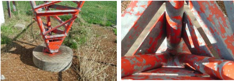
Figure 12. Details of Ashland foundation and shear pin.
