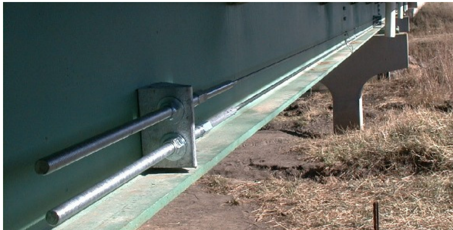
(c) Completed installation of exterior CFRP bars in west end span
