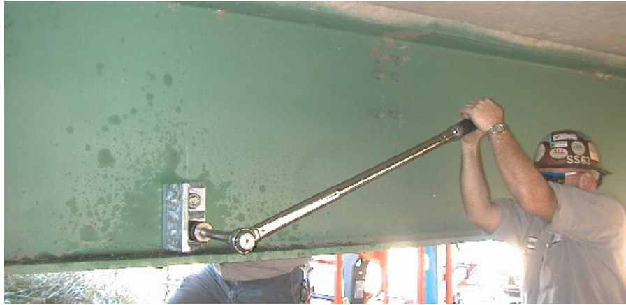
(a) Installation of anchorage assembly
