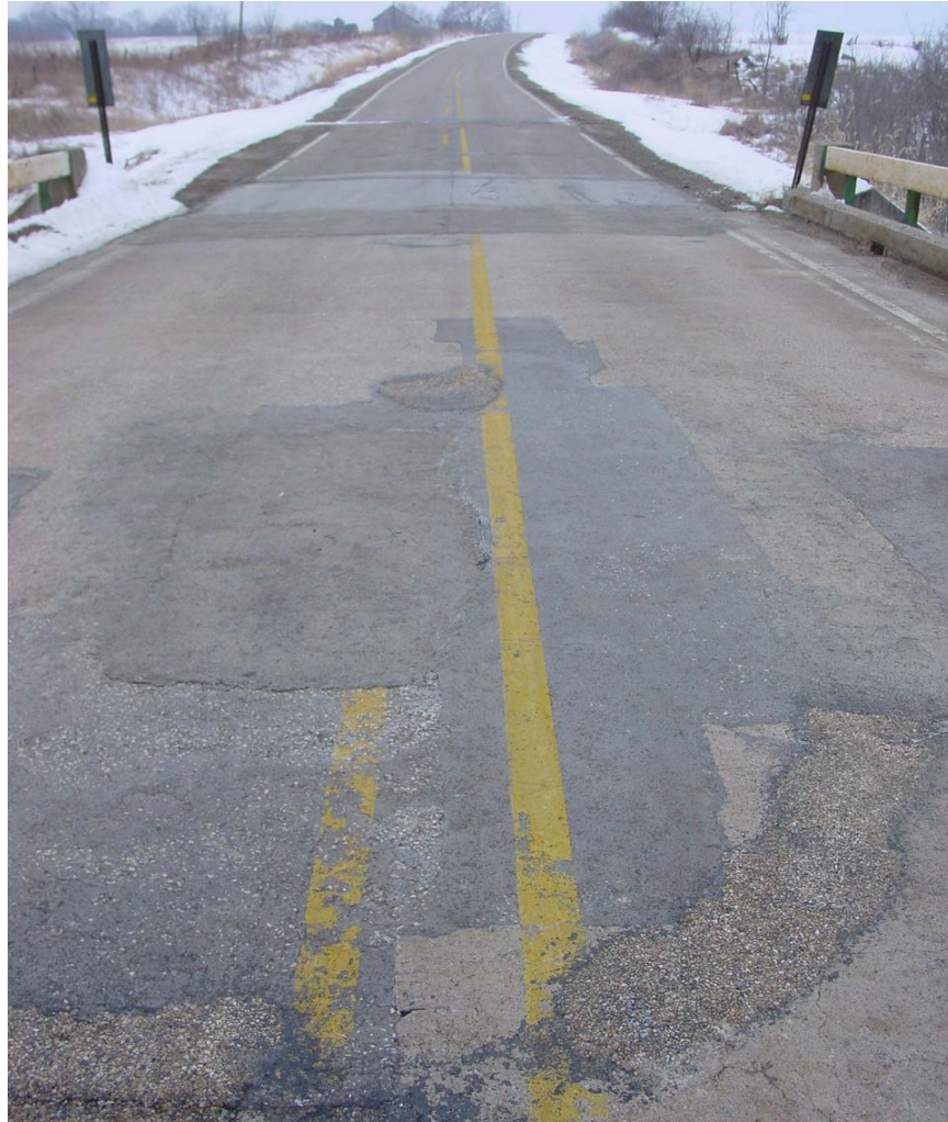
FIGURE 3 The Tama County Bridge to be used for the First Known Steel Free Deck in the United States.
