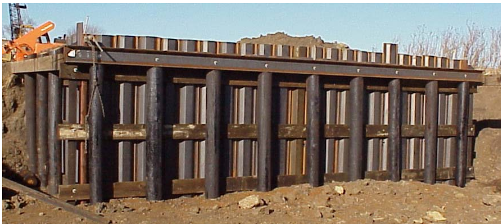
(c) Abutment under construction
