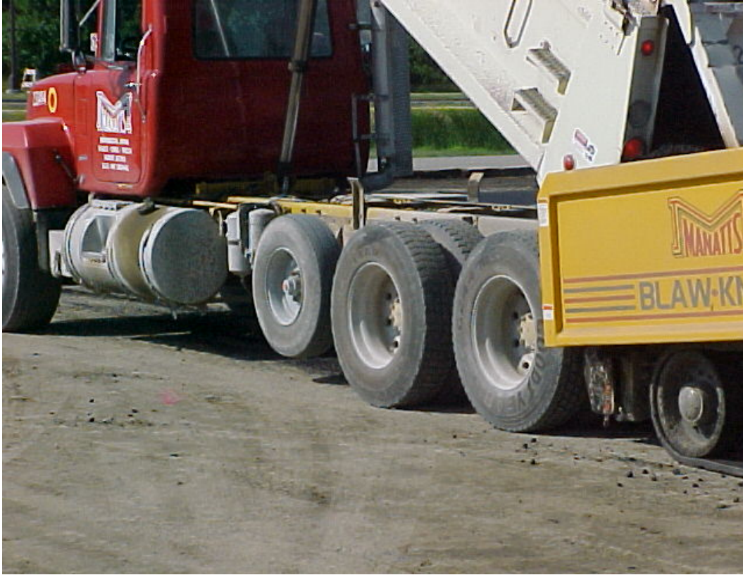
FIGURE 3 Newly Constructed Paving Platform
