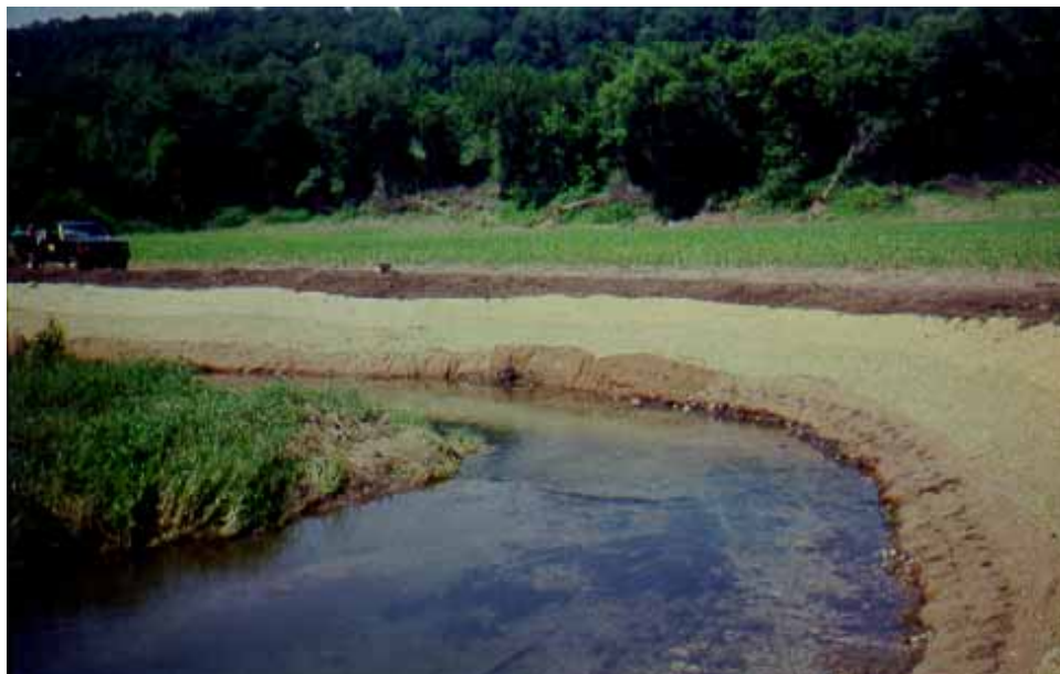
Figure 1. Streambank that has been graded and seeded using a natural fiber blanket containing seed
