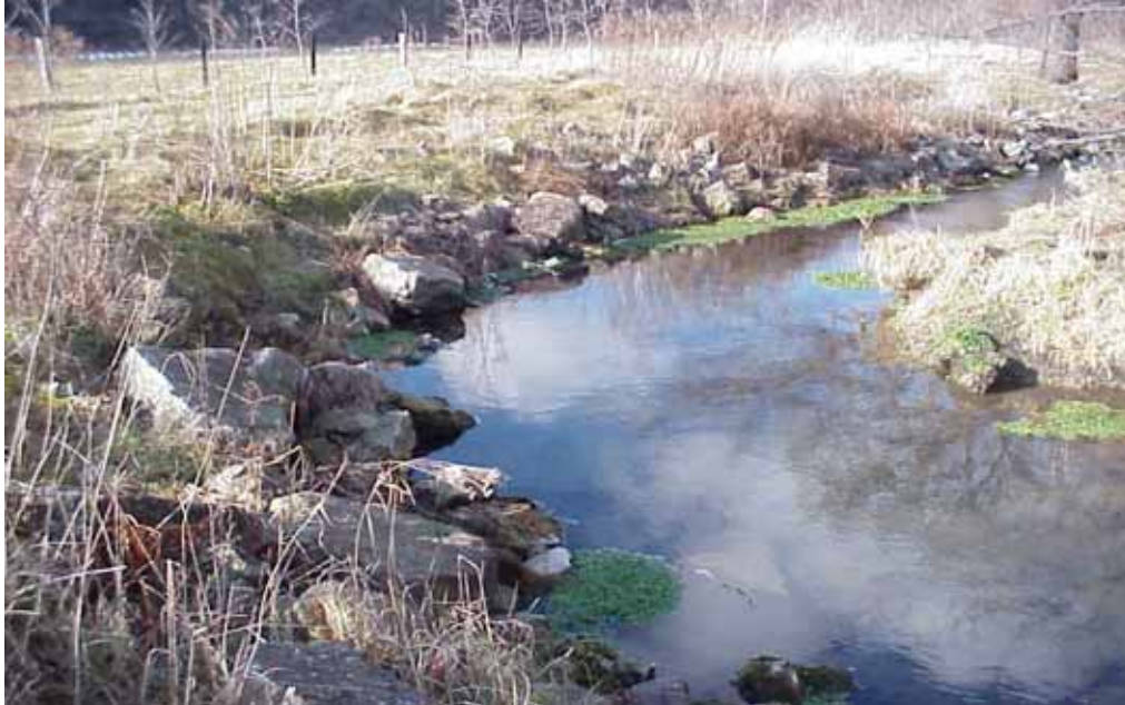
Figure 20. Riprap along the bend of a stream with vegetation between the rocks
