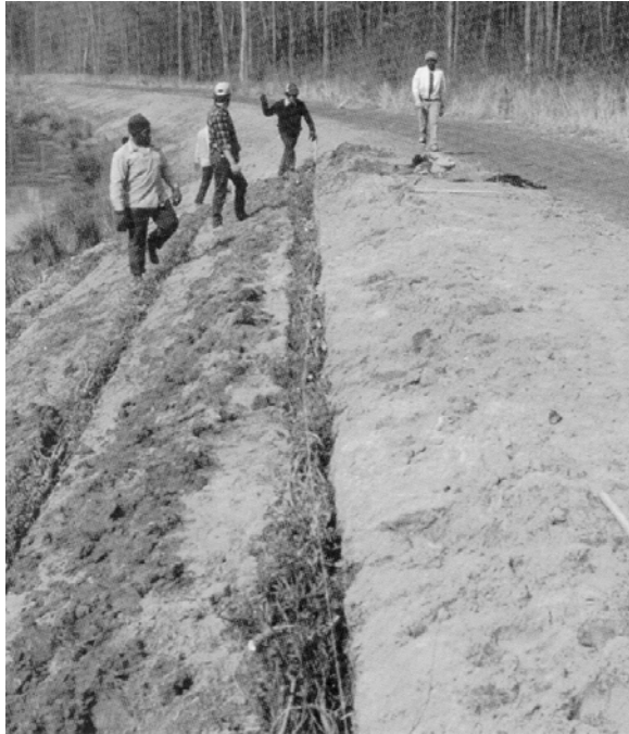
Figure 8. Live fascine placement
