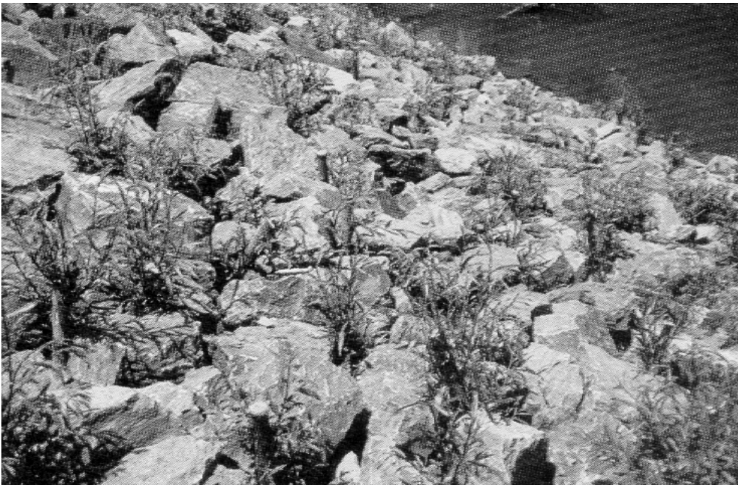
Figure 6. Joint planting system installation
