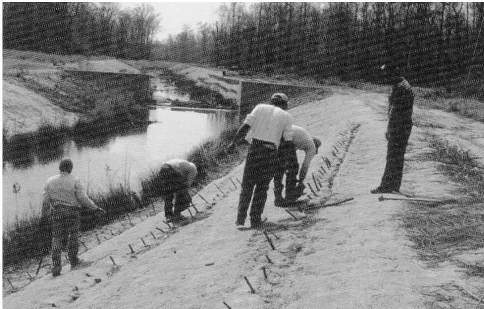
Figure 9. Live fascine stake network
