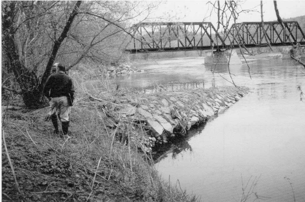
Figure 22. Stream jetty placement for bridge protection
