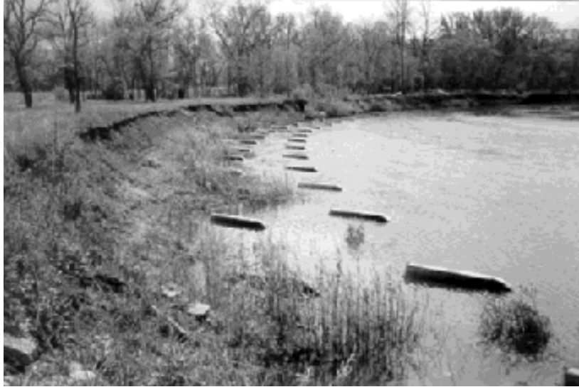
Figure 26. Replacement of sediment on bank from Vanes
