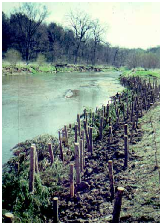
Figure 17. Willow posts on a streambank
