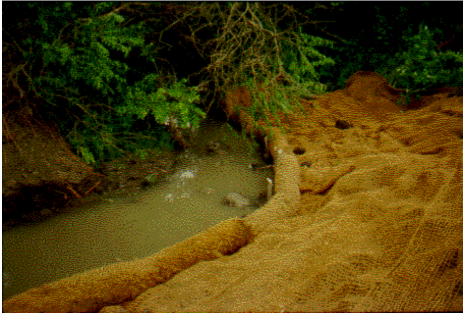
Figure 15. Coconut roll staked to bank with coconut fiber fabric across slope to protect exposed soil
