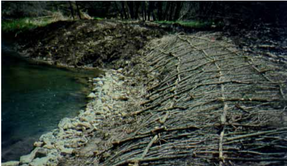
Figure 11. A brushmattress with riprap at the toe of the slope
