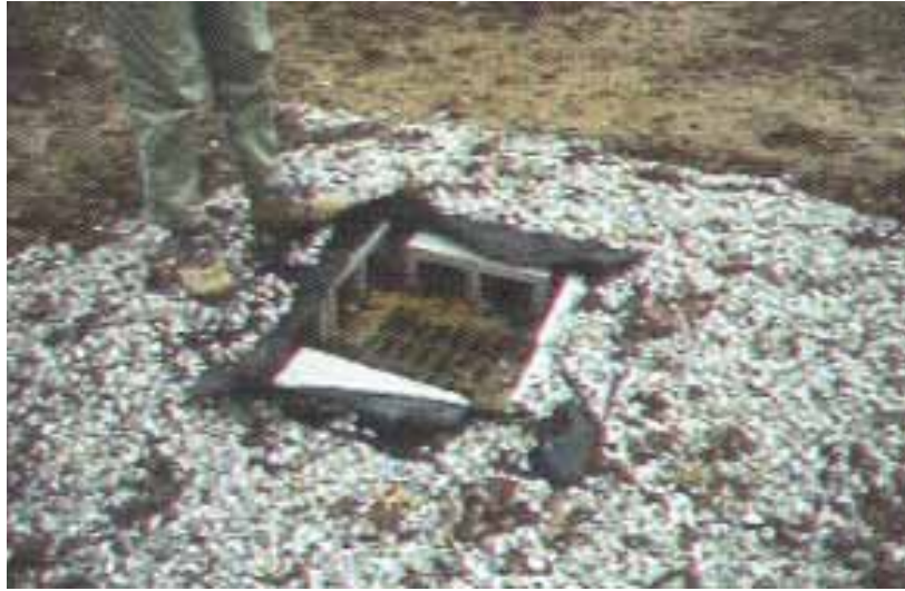
Figure 3.14. Inlet protection (Source: Minnesota DOT)
