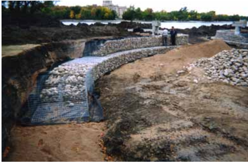
Figure 3.13. Gabion (Source: Modular Gabion Designs)
