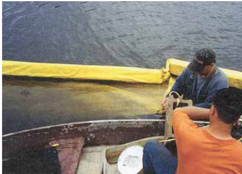
Figure 3.11. Flotation silt curtain (Source: Minnesota DOT)
