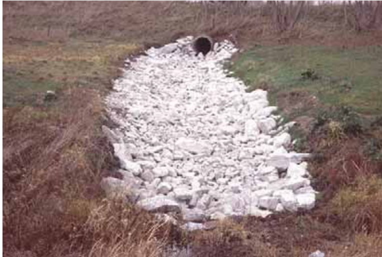
Figure 3.10. Energy dissipator (Source: Iowa DOT)
