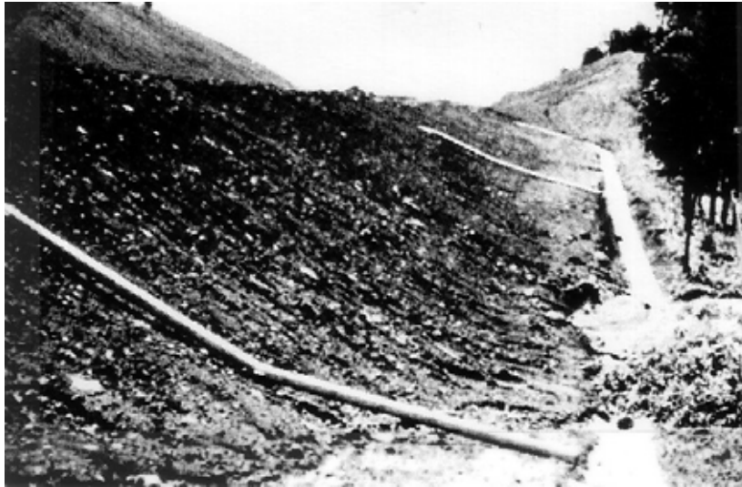
Figure 3.9. Temporary slope drain (Source: Department of Civil, Construction, and Environmental Engineering, Iowa State University)
