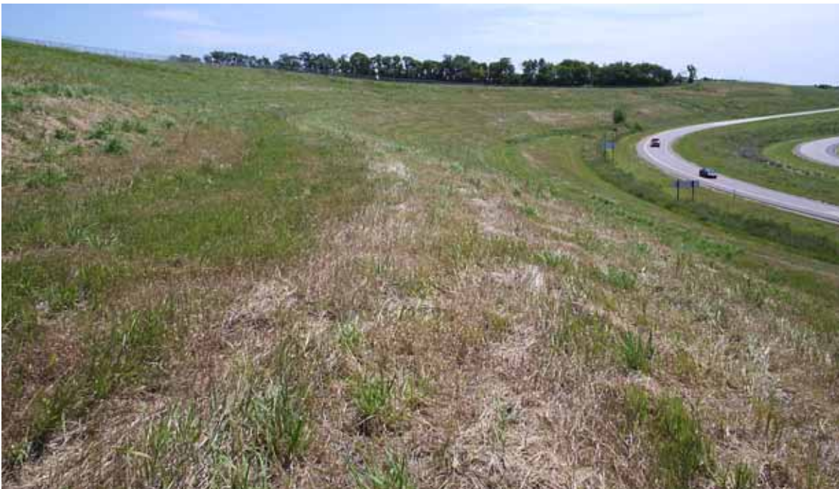
Figure 3.3. Bench cut, interchange application (Source: Department of Civil, Construction, and Environmental Engineering, Iowa State University)
