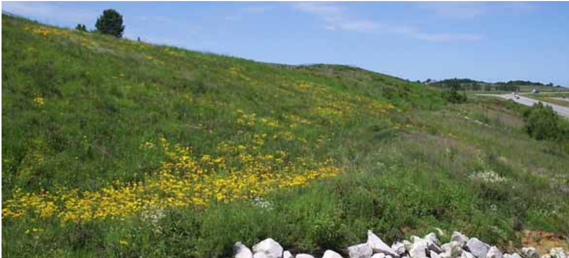
Figure 3.1. Bench cut, upper level (Source: Department of Civil, Construction, and Environmental Engineering, Iowa State University)
