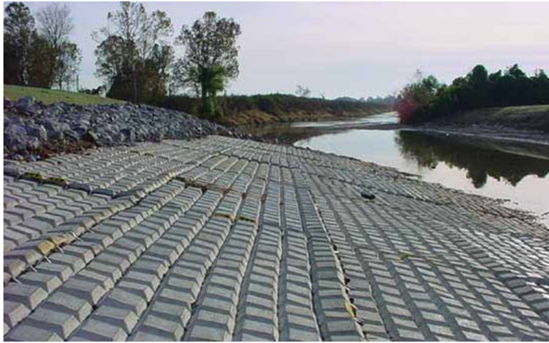
Figure 3.31. Streambank protection (Source: International Erosion Control Association)
