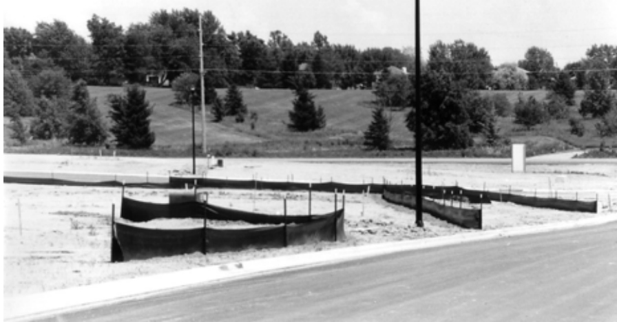
Figure 3.29. Silt fence sediment barrier (Source: Department of Civil, Construction, and Environmental Engineering, Iowa State University)
