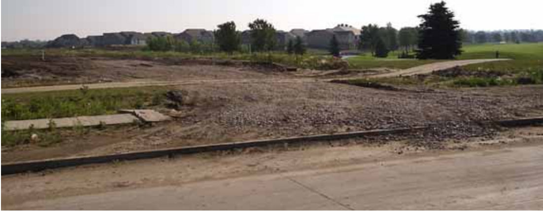
Figure 3.26. Temporary stabilized construction entrance to construction site (Source: Department of Civil, Construction, and Environmental Engineering, Iowa State University)
