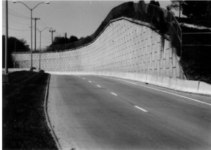
Figure 3.25. Retaining Wall (Source: Department of Civil, Construction, and Environmental Engineering, Iowa State University)
