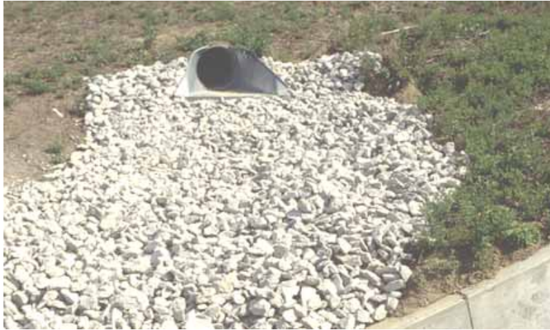
Figure 3.24. Rock outlet protection (Source: Iowa DOT)
