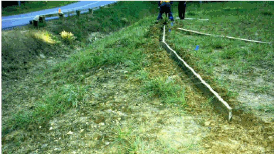
Figure 3.23. Level spreader installation (Source: William B. Umstead State Park)
