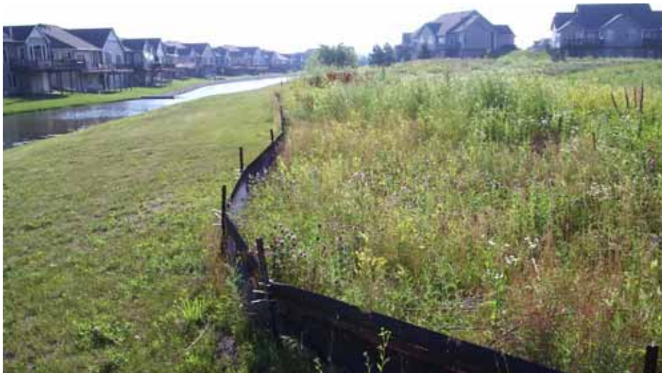
Figure 2.22. Urban filter strip (Source: Department of Civil, Construction, and Environmental Engineering, Iowa State University)
