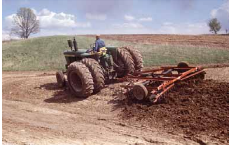
Figure 2.19. Surface roughening by disking (Source: Iowa DOT)
