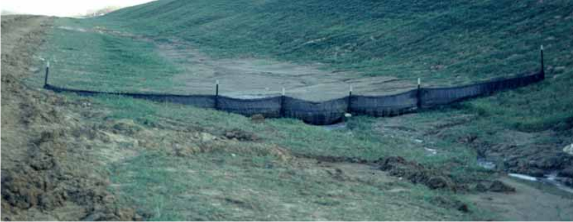
Figure 2.10. Silt fence (Source: Iowa DOT)
