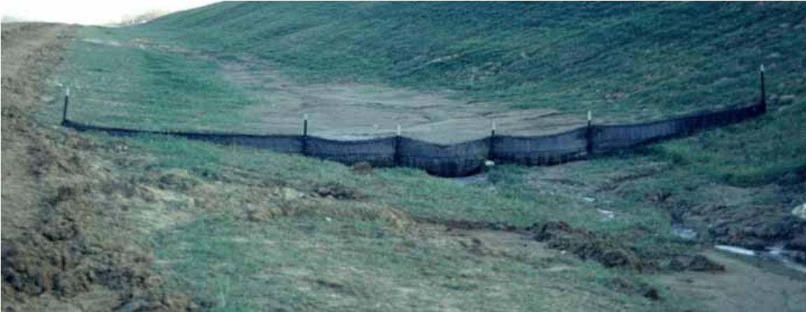
Figure 2.10. Silt fence (Source: Iowa DOT)
