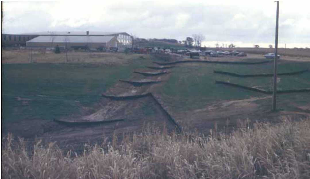
Figure 2.14. Proper silt fence installations (Source: Iowa DOT)
