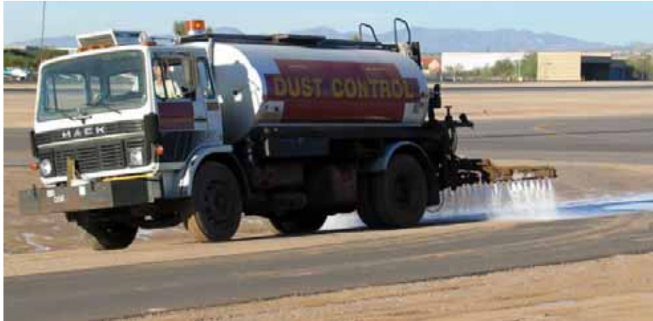
Figure 2.5. Truck-mounted dust-control applicator (Source: http://soiltac.com/Photo_Gallery.html )
