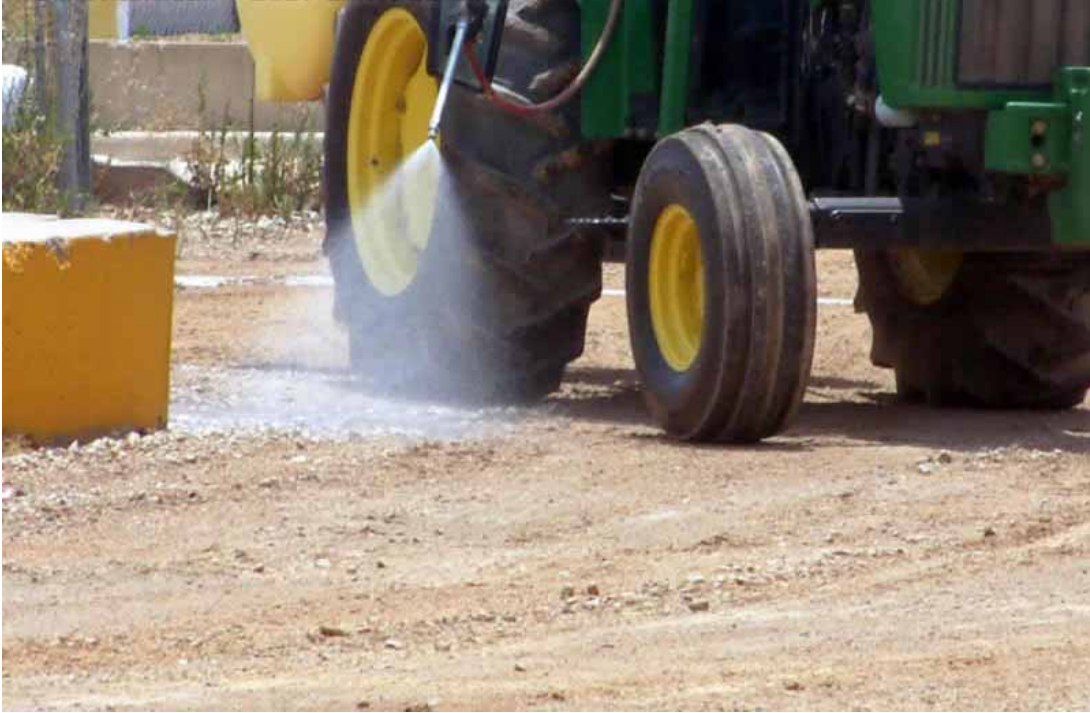
Figure 2.6. Manual dust-control applicator (Source: http://soiltac.com/Photo_Gallery.html )
