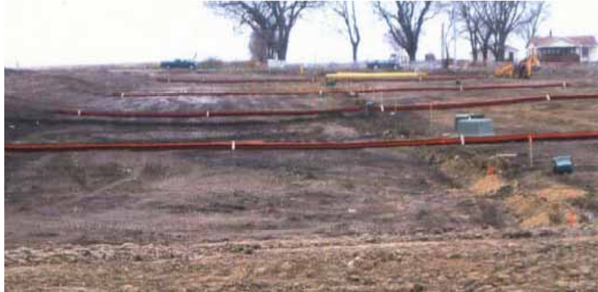
Figure 2.24. Compost filter tube (Source: SUDAS Design Manual)
