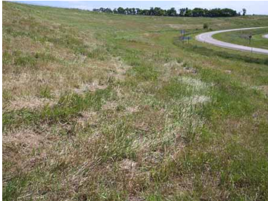
Figure 1.11. Diversion dike and swale combination (Source: ISU/CCEE)
